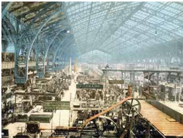
Galleria delle macchine. Expo 1900 Parigi. https://commons.wikimedia.org/wiki/File:Interior_of_exhibitions_building,_Exposition_Universal,_Paris,_France.jpg
